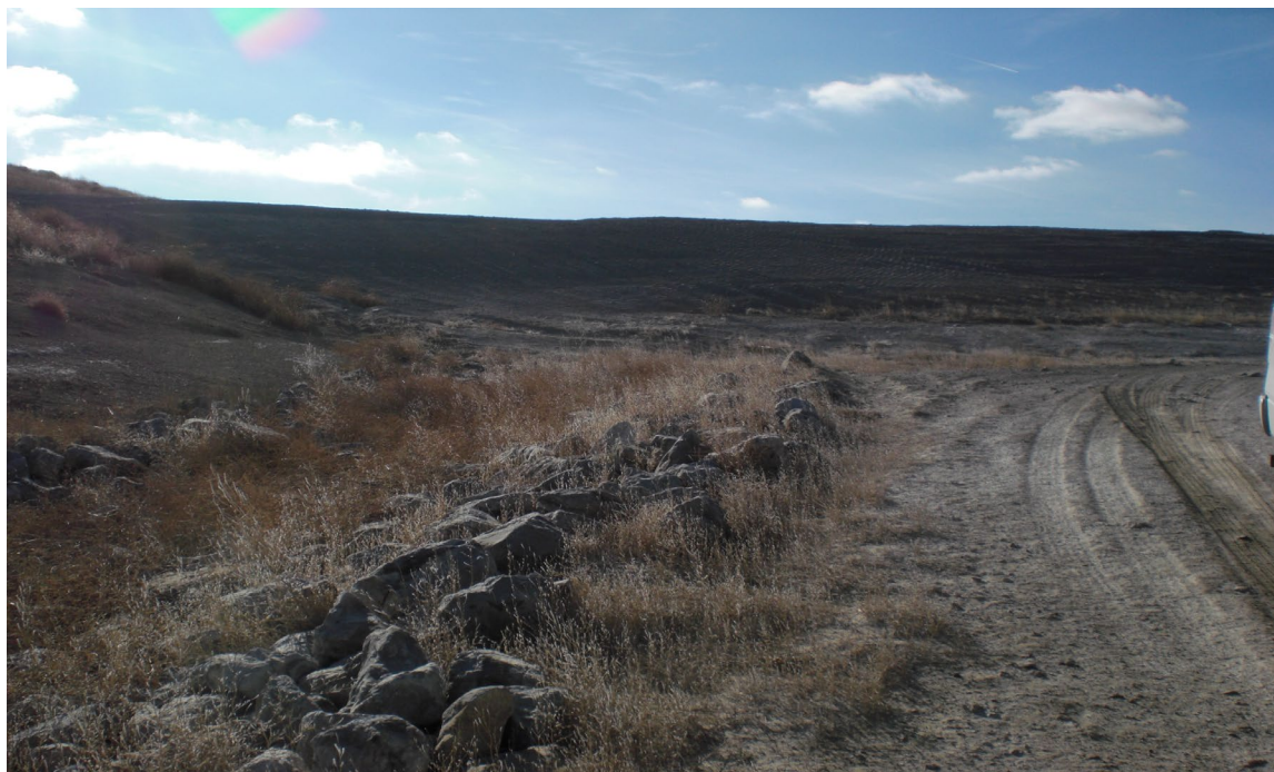
Photo 3: Contact water ditch for Landfill looking west
