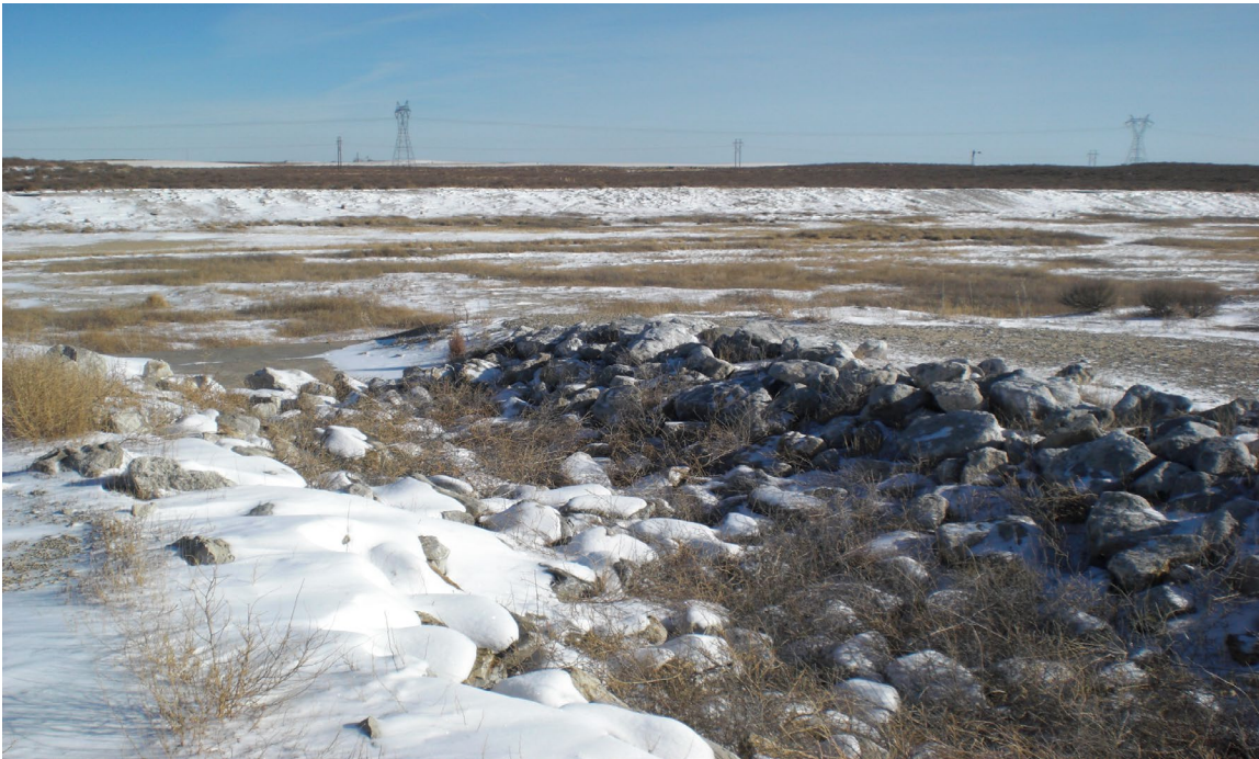
Photo 4: East end of contact water ditch to evaporation basin
