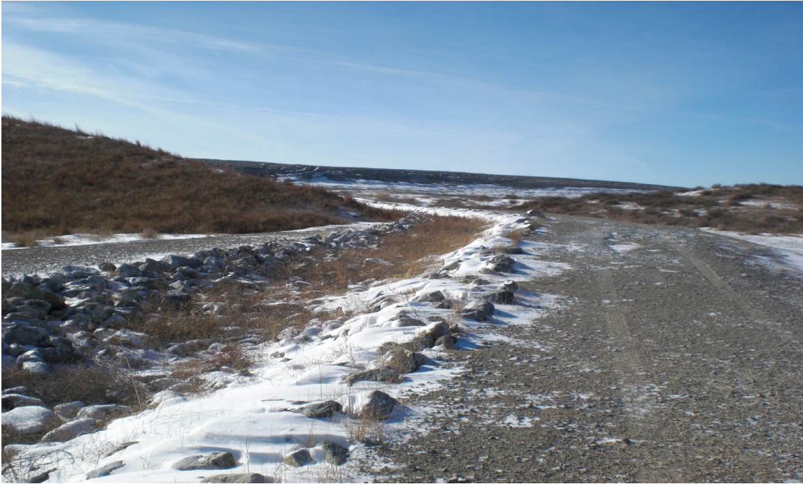
Photo 3: Contact water ditch for Landfill looking west
