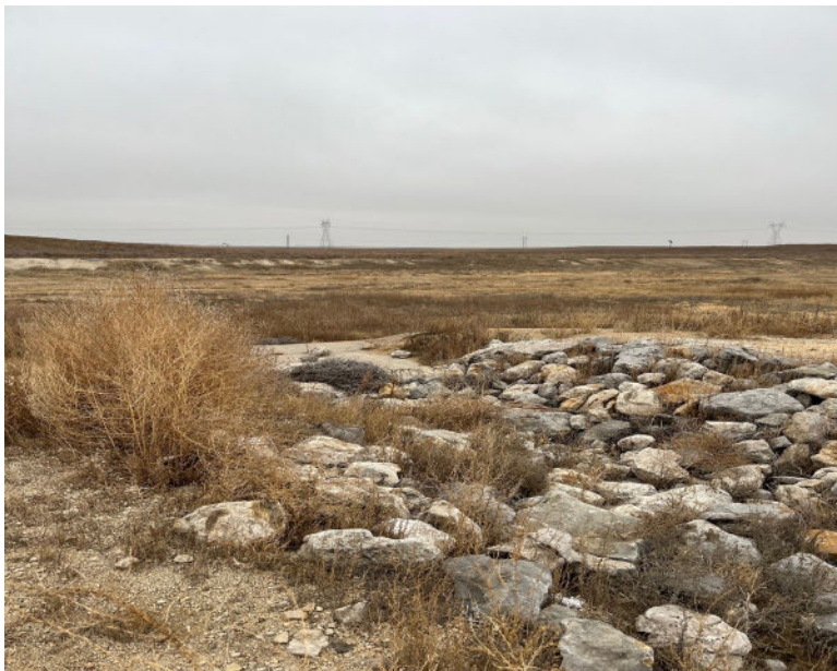
Photo 3: Contact water ditch for Landfill looking west
