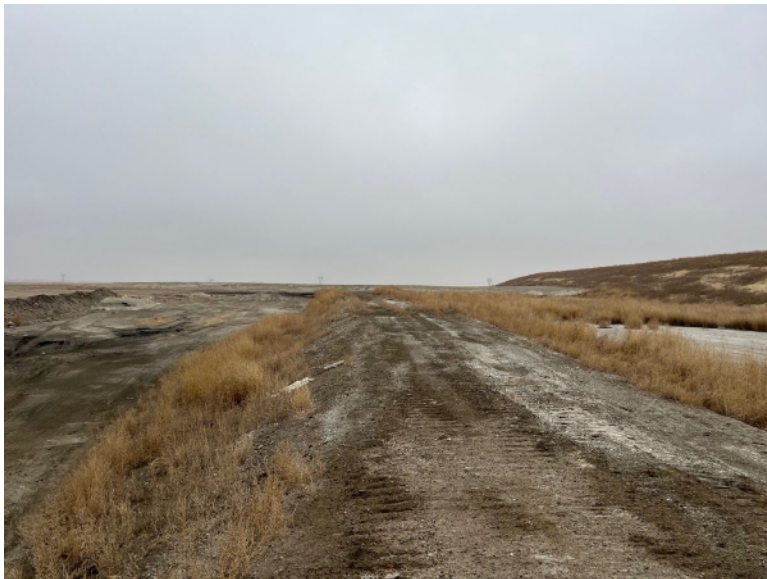
Photo 1: Entrance Road to Phase 3A
