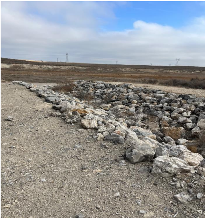
Photo 4: East end of contact water ditch to evaporation basin
