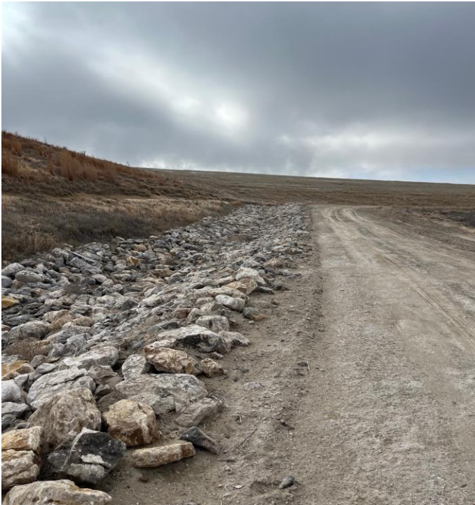
Photo 3: Contact water ditch for Landfill looking west
