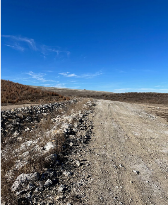
Photo 3: Contact water ditch for Landfill looking west
