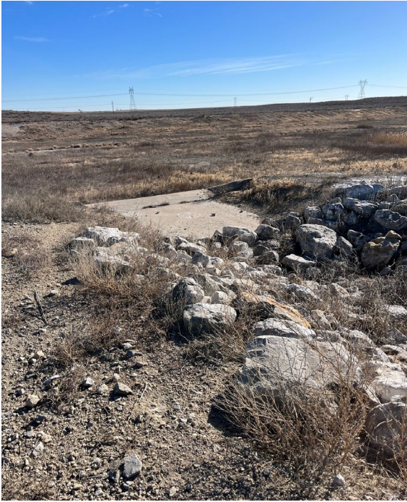
Photo 4: East end of contact water ditch to evaporation basin
