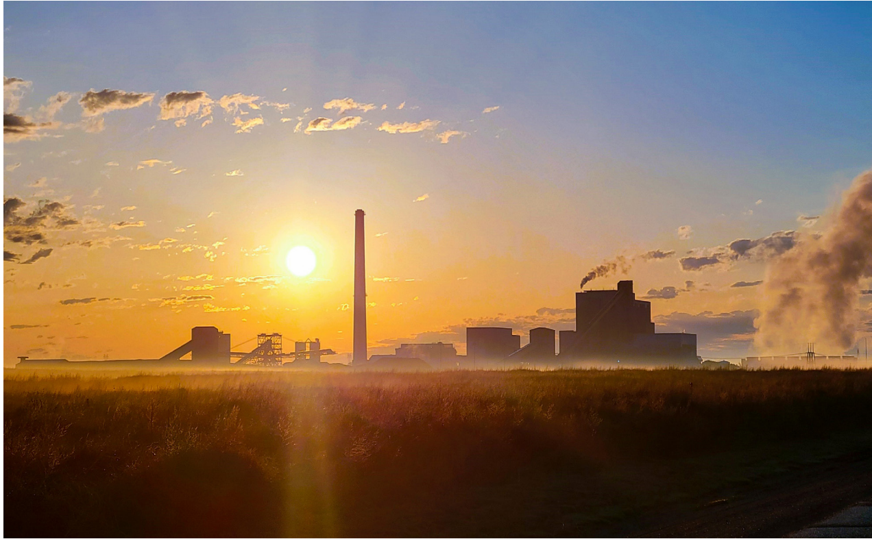
Sunrise at Holcomb Station, taken by Sunflower Generation Technician Brandon Smith.
