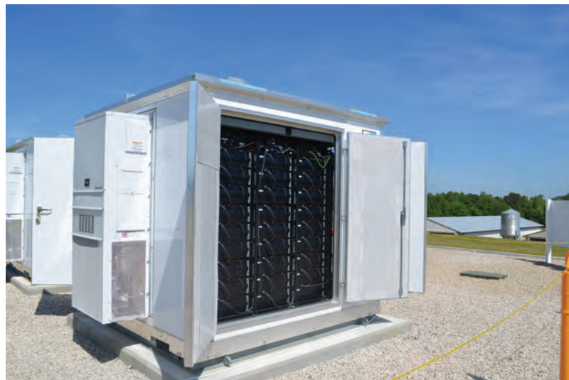
Energy storage plays a crucial role in incorporating renewable energy into our electric grid. Solar and wind energy are weather-dependent, so when energy demand is low, storing the excess energy makes it possible to use it later when demand is higher. This 250 kW/735 kWh battery storage facility is owned by North Carolina's Electric Cooperatives, in partnership with South River EMC. Photo Source: North Carolina's Electric Cooperatives.
