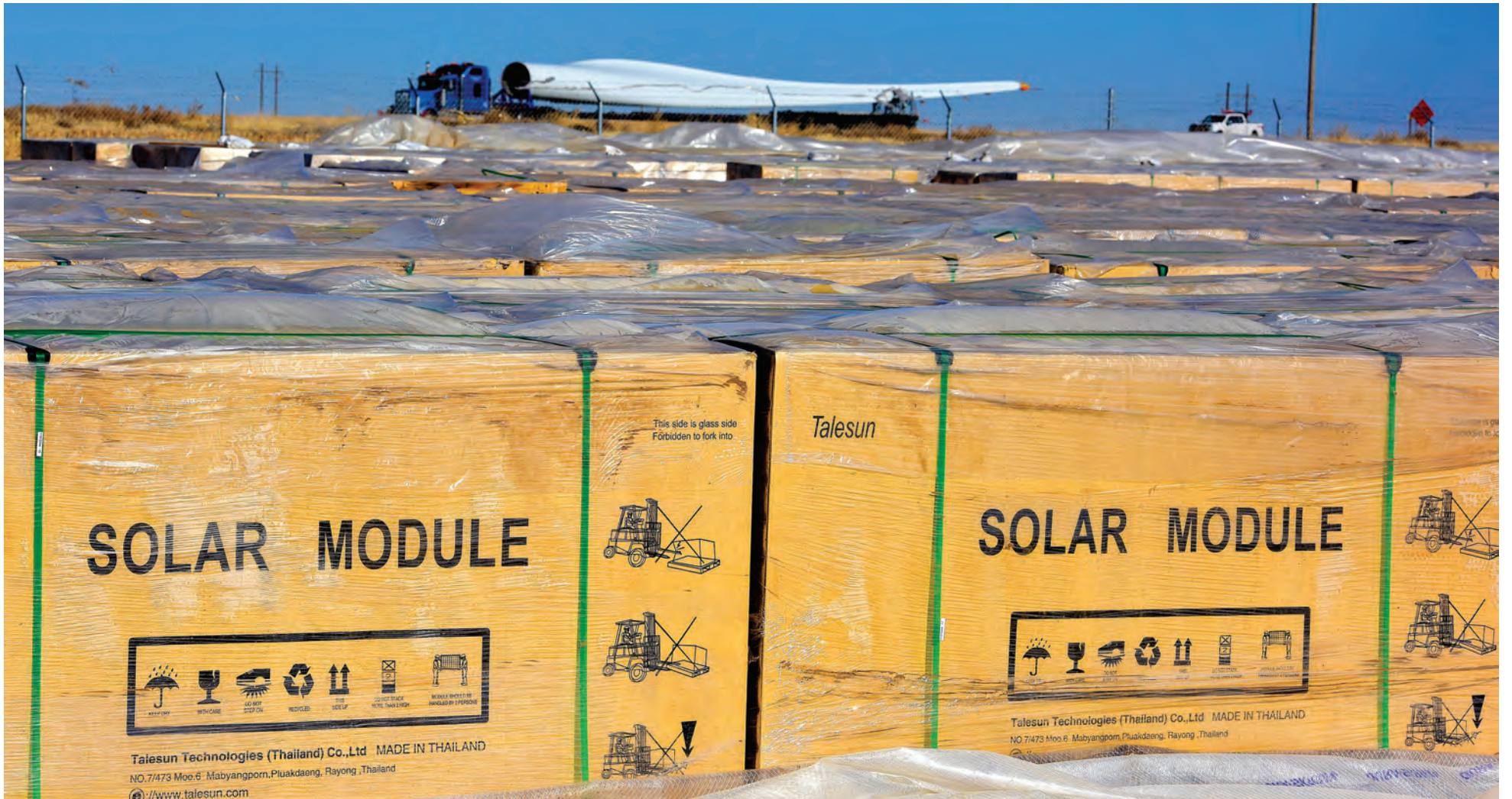
Harnessing Mother Nature creates diversified energy generation opportunities. Solar panels sit in a box ready to be installed at the Johnson Corner Solar Project in January 2020 in Stanton County while a semi-tractor delivers a blade to a wind farm under construction nearby.
