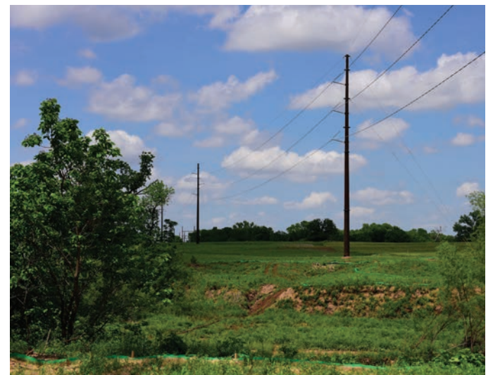
Top: Mid-Kansas developed the 110 MW Rubart Station with fast-start capable internal combustion units, allowing for quick response to market conditions. The facility became commercial in September 2014.
